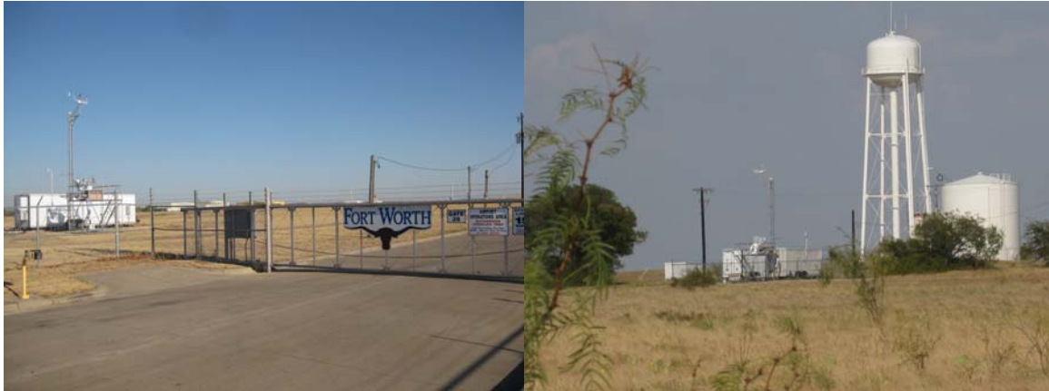
Figure 1. MOPS instruments installed and operating at the Fort Worth Northwest (left) and Eagle Mountain Lake (right) CAMS sites. These sites have collected multiple weeks of ozone production data that is currently being evaluated.
